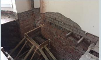
Much of the early work is focussed in the roof space and in the under croft below the ground floor. Both these spaces will contain much of the structural support required to remove the walls along with the mechanical and electrical equipment for the building.
